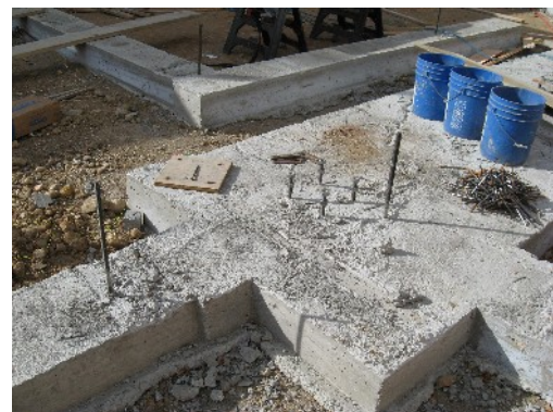
FIG 2: ANCHOR BOLTS AND HOLDDOWN ANCHORS CAST IN PLACE.
