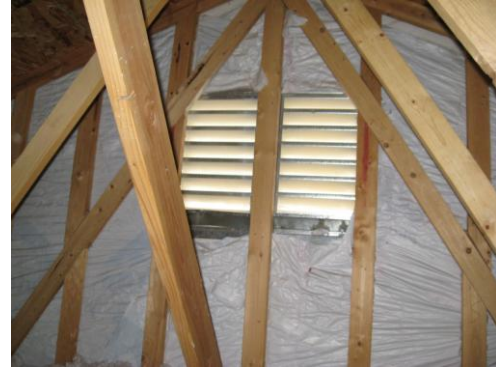
FIG 4: STRUCTURAL GABLE END.
