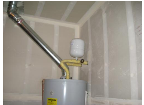
FIG 5: WATER HEATER, STRAPS NOT SHOWN.
